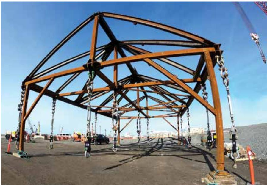
Straightpoint load cells were added to a custom-built lifting frame. Under the frame were a total of 82 55-ton shackles, 14 Crosby 2.75" turnbuckles, and four equalizer plates, in addition to the load cells.
