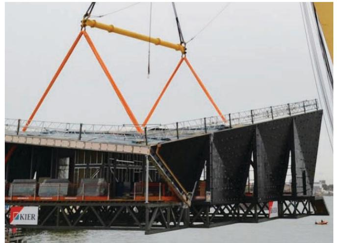
**Lift with load centered correctly.**
