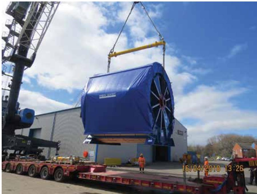
The Modulift beam was required to lift the dual reels that contained two mooring lines. An additional spreader beam and rigging was required for the spare single reel. The two MOD 70 spreaders were supplied at 3.11m-wide with custom length struts.
