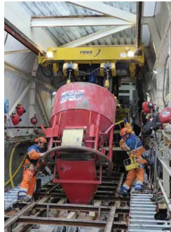
A Rowa employee (right) can be seen wearing the bellybox remote control that operated the four GIS hoists on the machine above.
