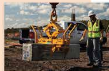
On the job at Florida's Orlando International Airport
